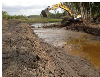
Breaking through the bund - 70yrs of sediment and bund cleared.
