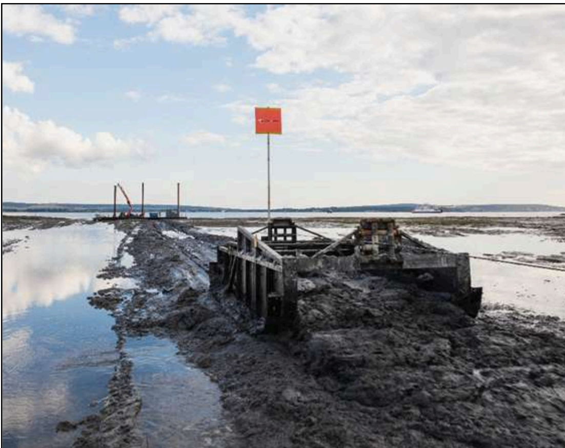
Saltmarsh Restoration Drag Box bringing mud onto Boiler Marsh. Courtesy of Lymington Harbour Commissioners.
